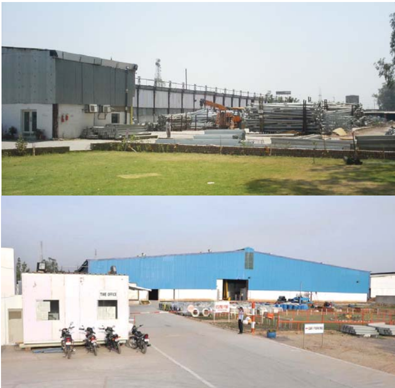
Synergy Telecommunications facilities in Nalagarh in Himachal Pradesh and Mohali in Punjab.
