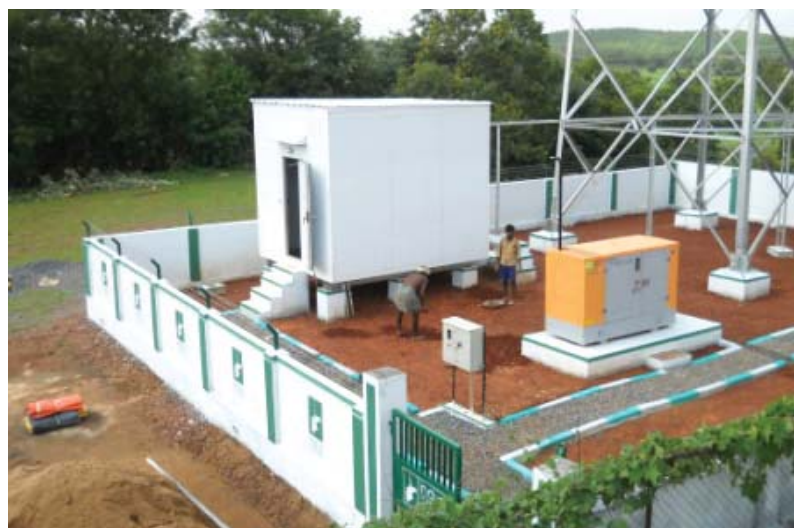
A cell site under construction.
