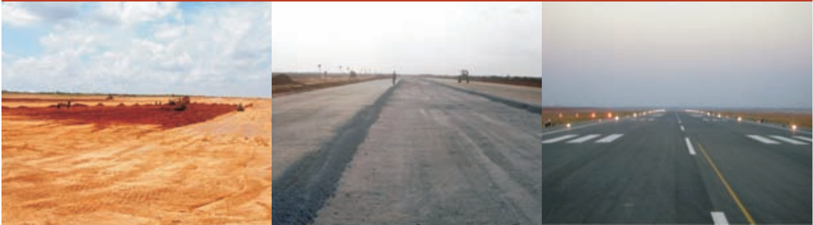
The runway in 2005, 2006 and after completion in 2008
