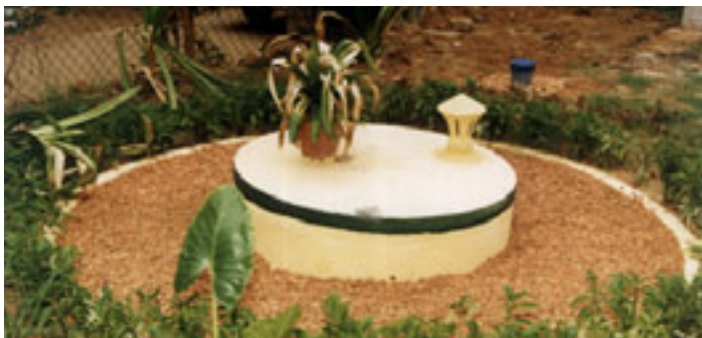
A surface level recharge structure in Chennai that stores rainwater and lets it percolate underground.
