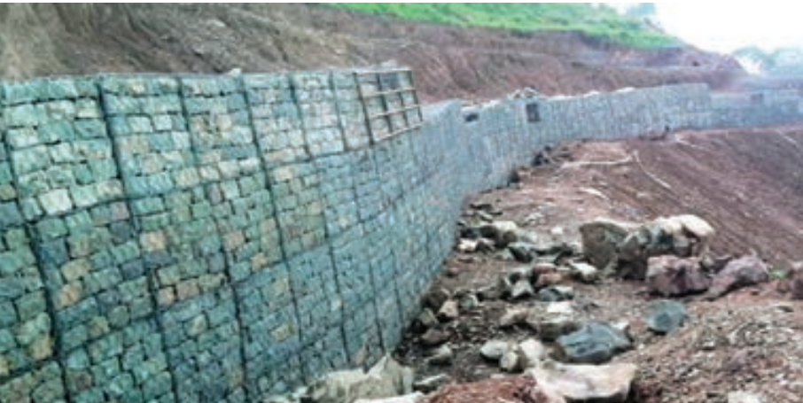
A wall made of stacked and stone-filled gabions tied together with wire, instead of roller-compacted concrete retaining walls. (right) Snowfall at the worksite.
