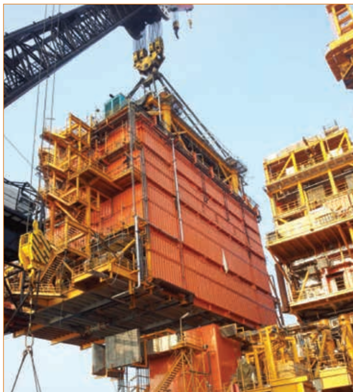
Installation of living quarter and process decks
