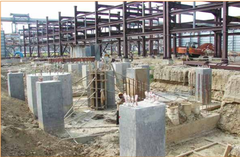
Pipe rack and foundation for technological structure at Butadiene Extraction Plant, Panipat
