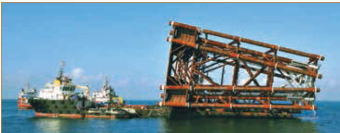
Jacket being sailed for installation to the offshore processing platform
