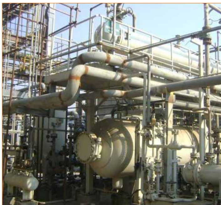
Butadiene refrigeration system in the Panipat refinery
