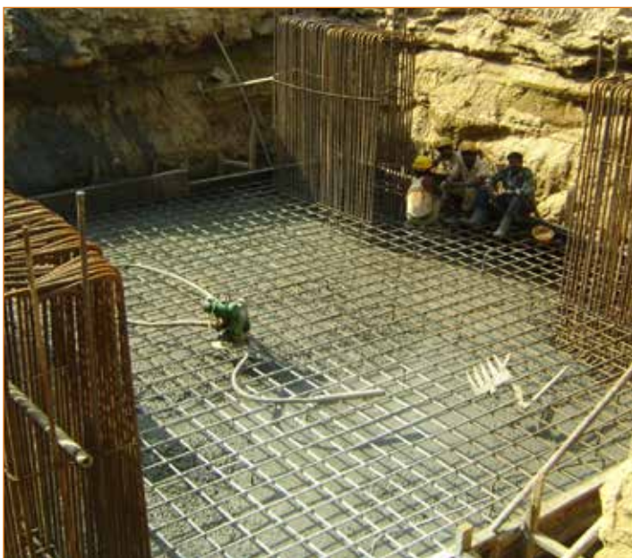
Shuttering works at the foundation of the butadiene extraction plant in Panipat
