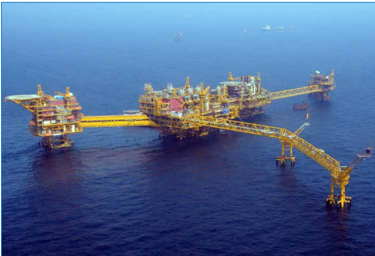
An aerial view of the massive Mumbai High North complex. This project achieved several 'firsts' for Indian offshore such as the largest jacket, heaviest load out, heaviest offshore lift, largest offshore living quarters module, and largest process platform.
