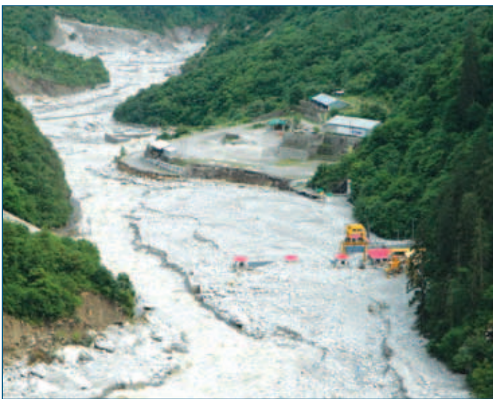
The Vishnuprayag dam that suffered extensive damage during the recent flood (Photo courtesy: MATU Jansangathan)
